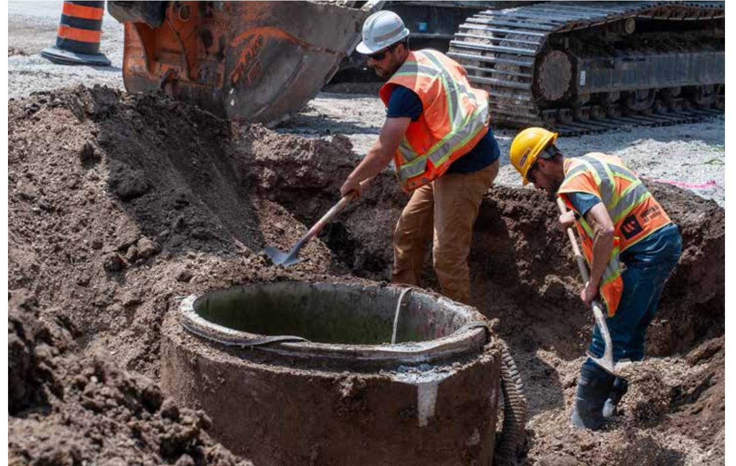
Kevin Karn and Troy McEwen work on replacing a culvert and catch basin on East Bayshore Road, near Owen Sound. Also on the job site that day was Jason Witte.
