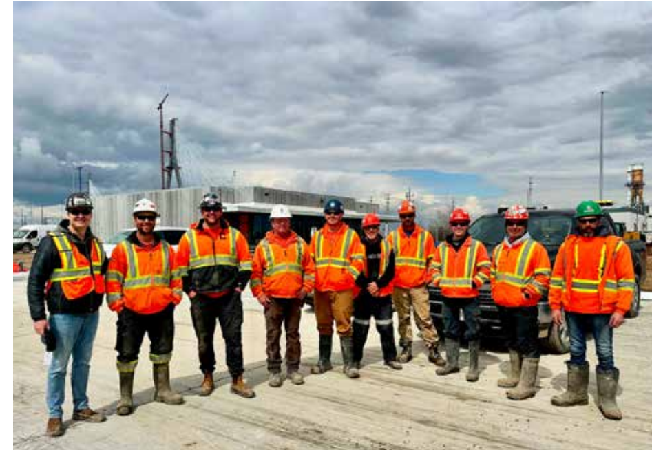
Local 1059 Business Rep Perry Thomas with members Colin Anderson, Avry O'Neil, Dave Guthrie, Brandon Robins, Jamie Graham, Tyler Rosborough, Creedyn Bragg, James Alves, and Joe Faria installing fencing at the Gordie Howe Bridge in Windsor
