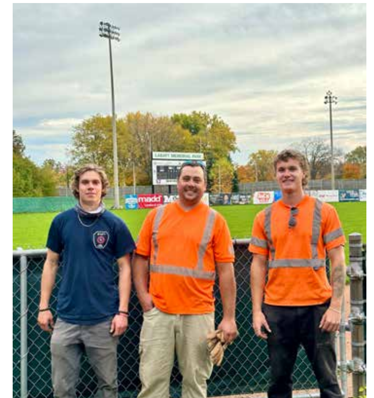
Apprentice Tanner Strain, Foreman Stephen Sloetjes, and apprentice Colton Kingswell installing updated lights for KWS Electric at Labatt Memorial Park
